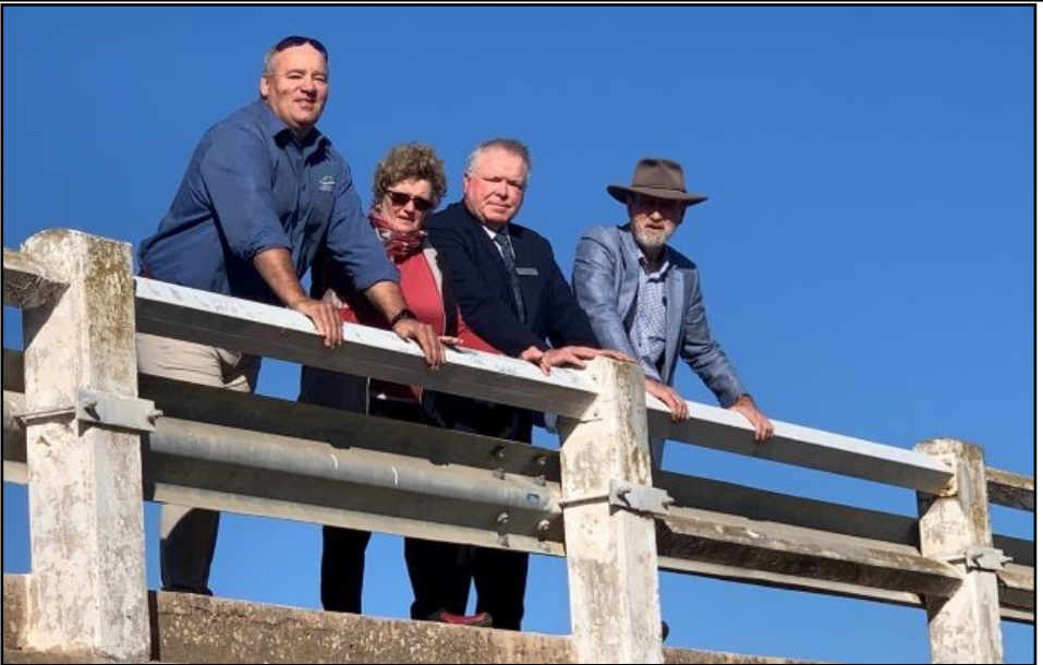
Mayor Mount Remarkable Council Phillip Heaslip, Northern Areas Councillor Denise Higgins, Mayor Northern Areas Council Ben Browne and Rowan Ramsey inspect the Pine Creek bridge.
